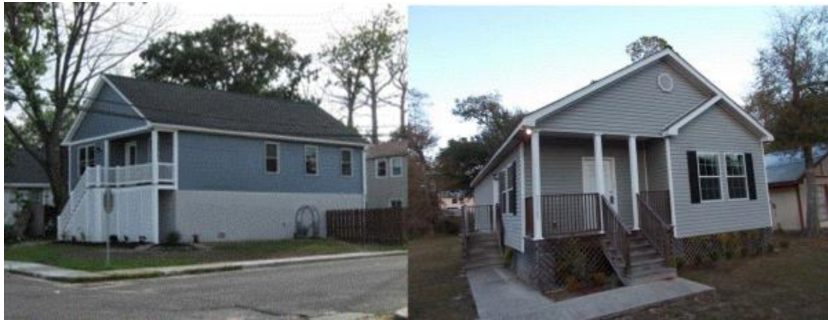
Figure 1 These homes have been elevated.
